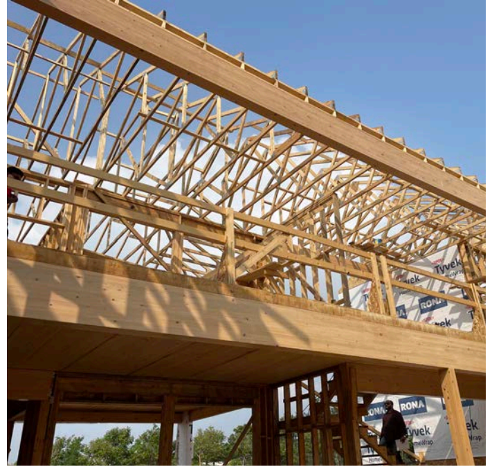
Second floor under construction | Credit: Canadian Wood India
