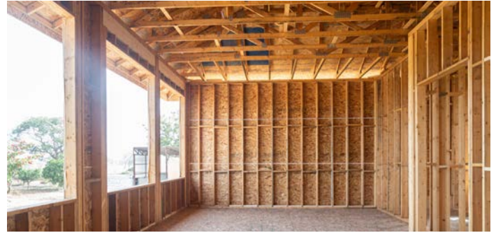
SPF wall framing and OSB sheathing | Credit: Canadian Wood India
