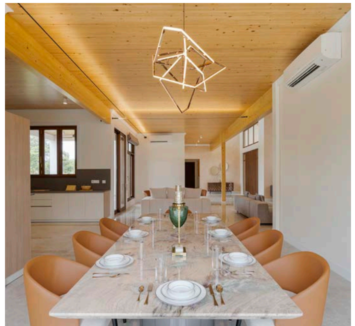
Dining area with exposed glulam beams and ceiling | Credit: Canadian Wood India
